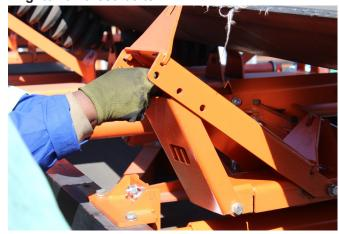
STEP 15: Install all of the idlers onto the frame.
