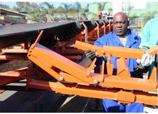
STEP 10: Secure tracker to the brackets that were installed earlier and fasten the bolts and nuts.
